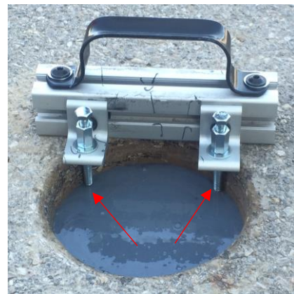
Fill core ONLY TO the bottom of the depth gauge extensions. Remove any excess adhesive before placing light to avoid messy overspill.
