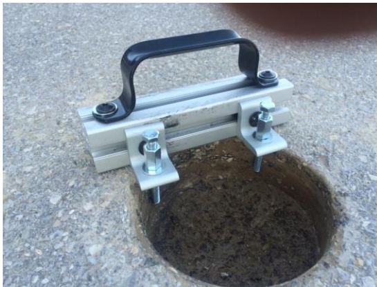
Place the Depth Guide in the core as a point of reference for proper adhesive fill Level. Proper depth of gauge is 35mm.
